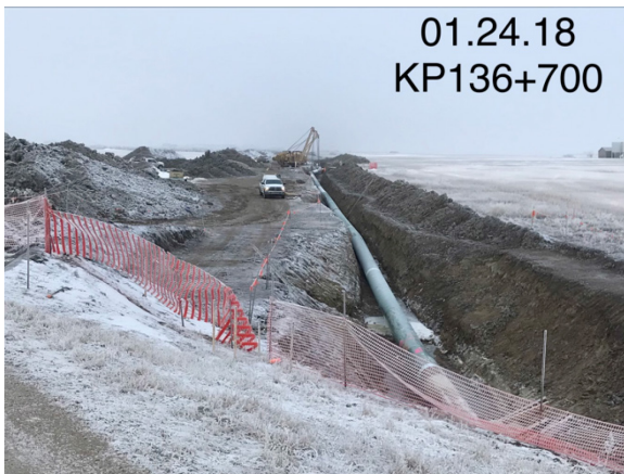
5. Tie-in ditch – Km 136+700 – Jan 24, 2018
