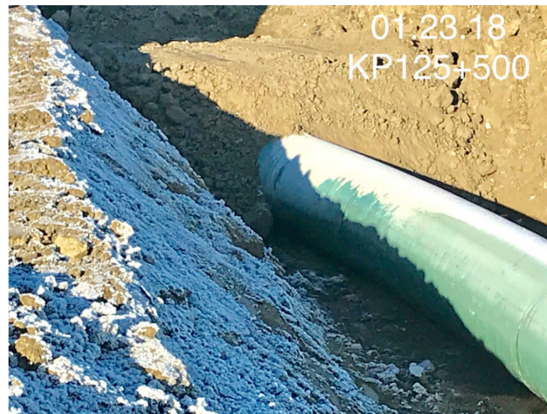
4. Chunk of dirt next to pipe – km 125+500 – Jan 23, 2018
