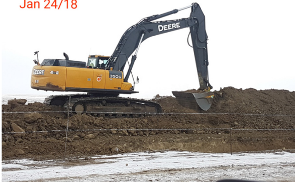
BACKFILL KP114+900 Jan 24/18
