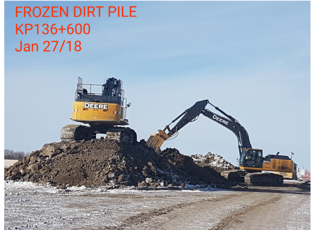
14. Frozen dirt pile – 136km+600 – Jan 27, 2018
