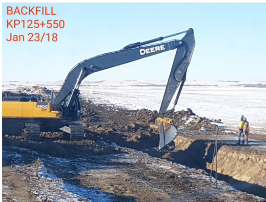
3. Backfill – Km 125+550 – Jan 23, 2018
