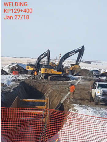
13. Welding– Km 129+400 – Jan 27, 2018
