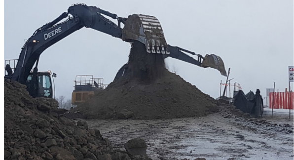
DIGGING KP124+100 Jan 25/18
