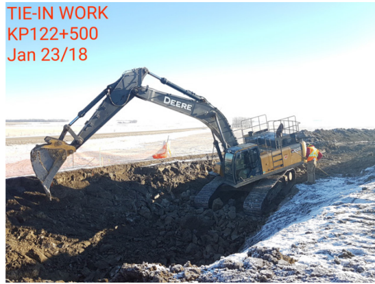
2. Tie-in – Km 122+500 – Jan 23, 2018
